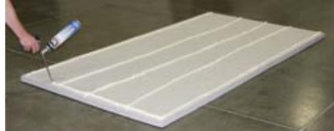
Apply Hilti or Touch 'n Seal All Seasons Foam on the back of the ECOCELL® blanket across the top and in vertical lines as pictured. Adhesive will adhere in 30 - 60 seconds and cure in 30 minutes.
