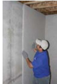
Align the seam of the blanket with the wall's edge or previously installed blanket. Work from the spacer\* to the ceiling to apply the blanket to the wall, pressing firmly.
