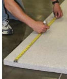
Start at a square corner of the room. Measure length and width of blanket needed for wall application. Then measure and mark blanket.
