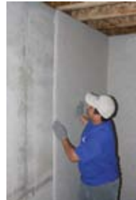
Unfinished room insulated with ECOCELL® blankets
