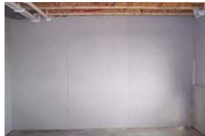
Unfinished room insulated with ECOCELL® blankets
