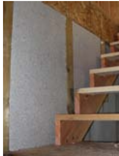
Unfinished room insulated with ECOCELL® blankets
